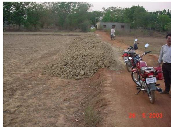
*Photographs showing poor earth work in embankment*
