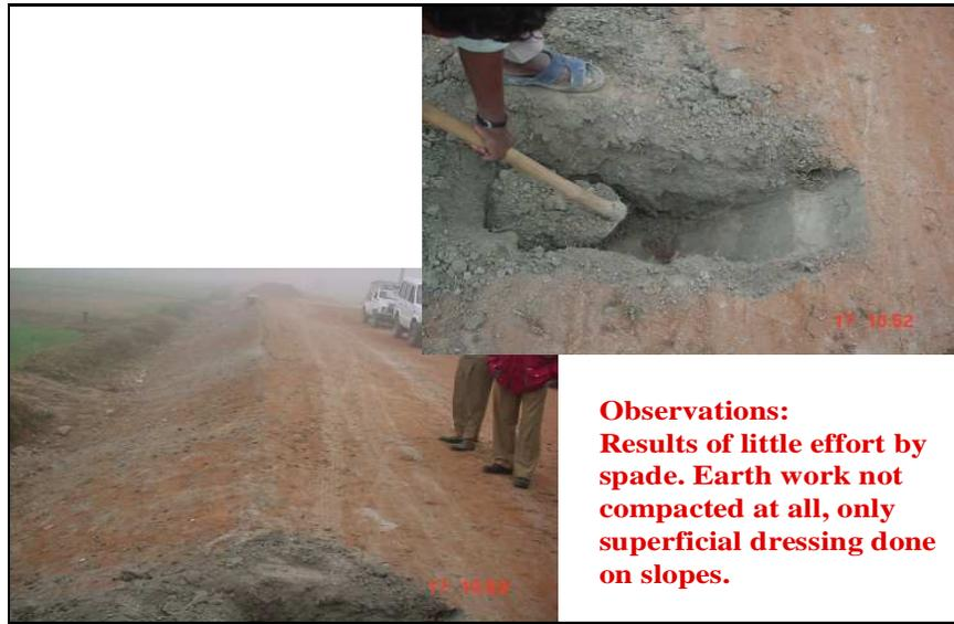
*Photographs showing poor earth work in embankment*
